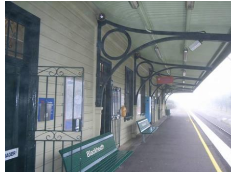
State – Blackheath Railway Station Group
