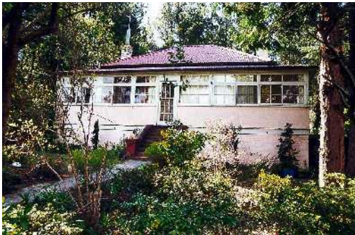
Local – Cottage at Blackheath
