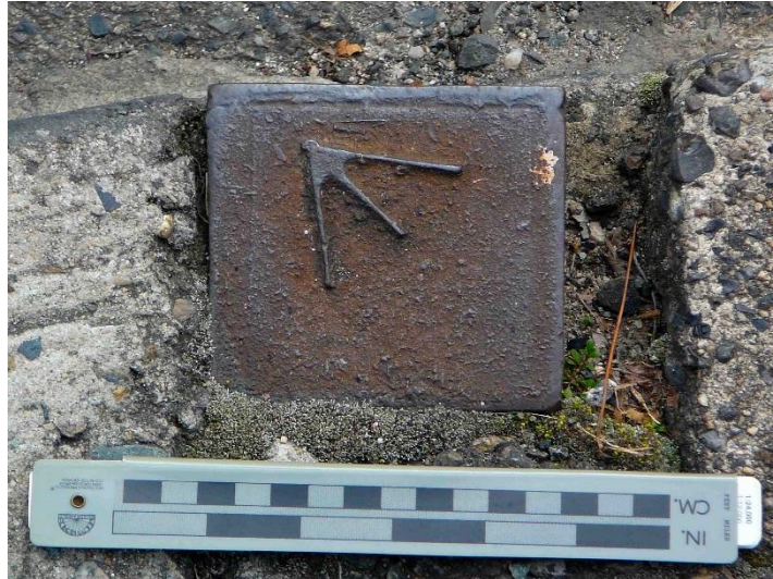
Figure 2. Alignment marker on the kerb of Station Street outside The Imperial Hotel, Mount Victoria. Photo: Peter Rickwood July 2011.
