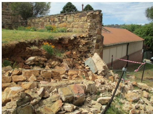
Emergency works – stone wall, Carcoar
