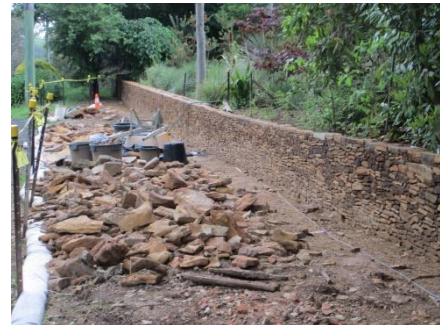
Under construction, Leura
