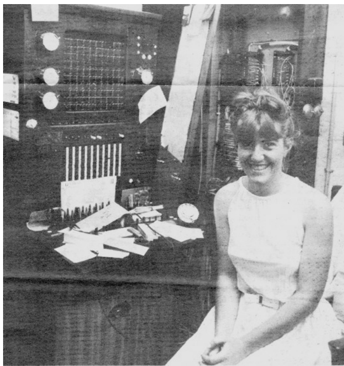
Sally Bailey, daughter of Mount Wilson manual exchange operator, Val Bailey, seated before the decommissioned 100 line operator assisted manual exchange board. The exchange was replaced by a 200 line fully automatic rural crossbar exchange.
