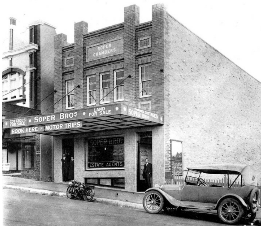
Figure 3. Soper Brothers store, Katoomba Street, Katoomba. (BMCCL LS IL 618).
