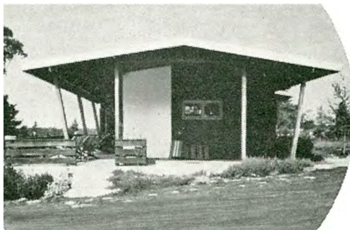
Figure 6. End elevation of the carport at Suvretta , Blackheath (Anonymous n.d.).
