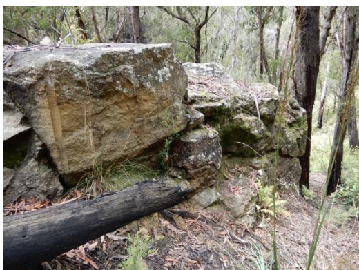
Evidence of blasting to create a cutting
