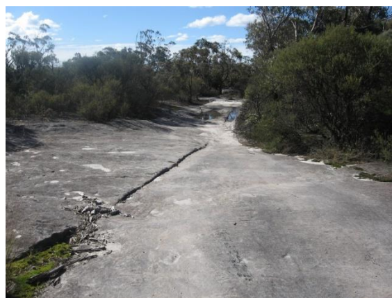
Rock drains near Woodford – on Cox's Road alignment
