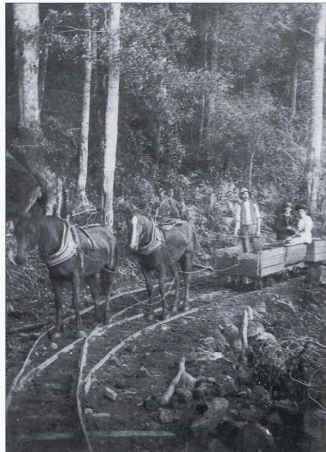
A horse tram on the line to Ruined Castle.
