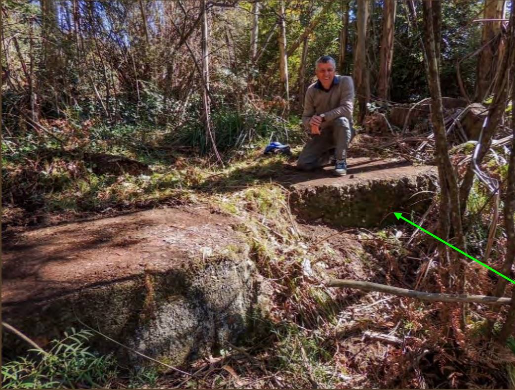
Here are the 2 concrete footings still on site. On the left the original turnwheel footing. On the right the clipwheel footing.
