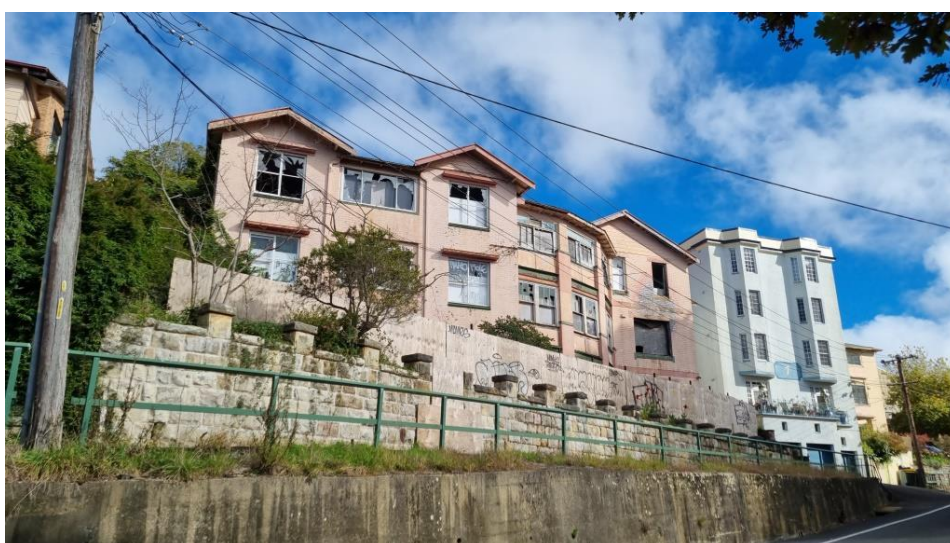
Views of the state of the building in May 2026
