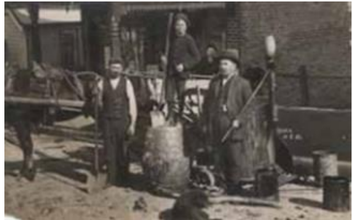
Road tarring gang in front of Fowler shop 1910
