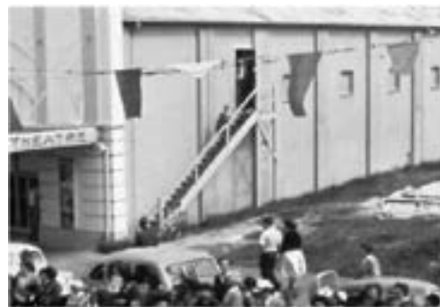
Stair to projection box
