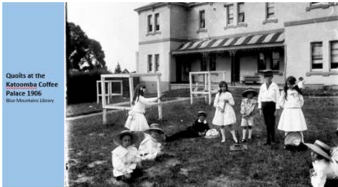
Figure 15: Quoits at the Katoomba Coffee Palace 1906
