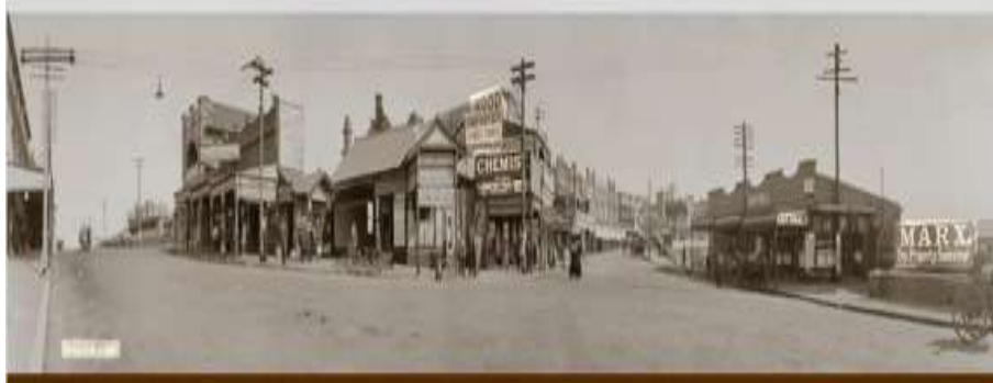
Figure 4: Main Street & Katoomba Street – centre of NYE activities
